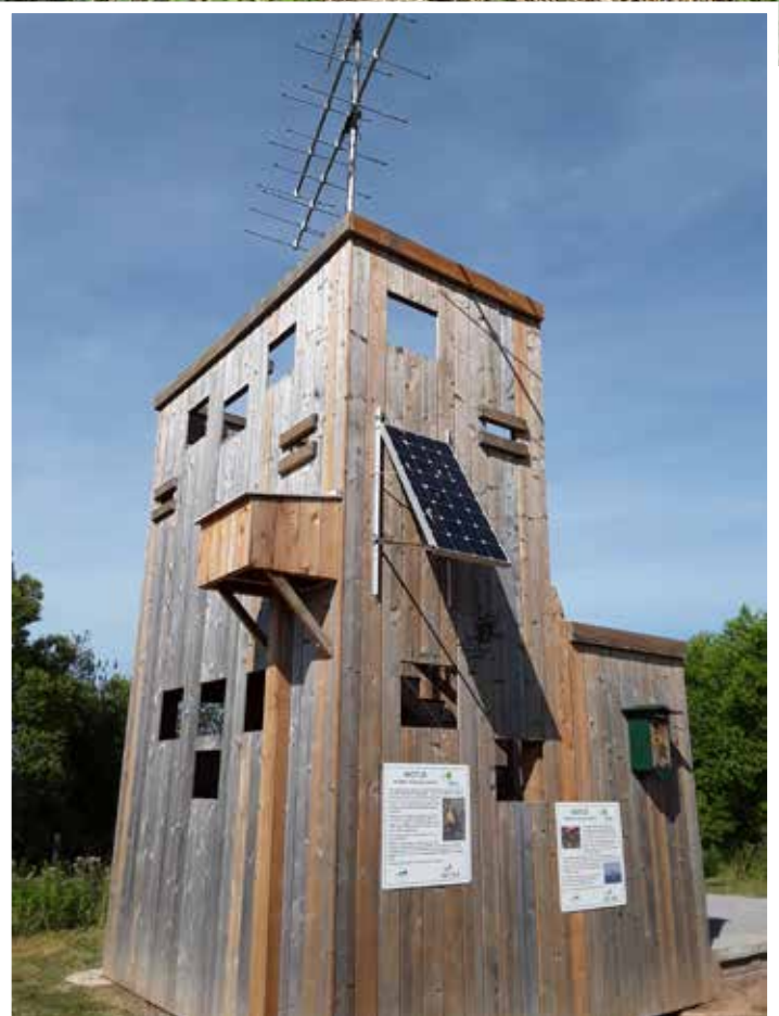
► The completed two-storey wildlife observation structure has a radio tracking tower that uses the specialized Motus program to collect data on migrating creatures.
